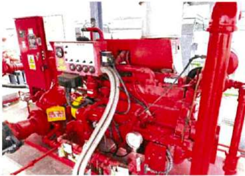
Diesel engine fire pump
