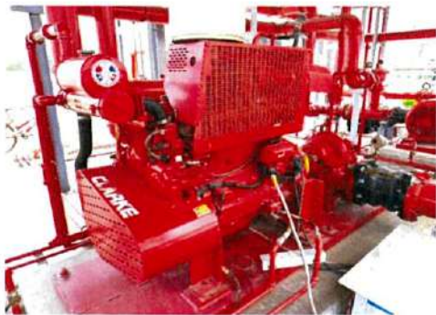
Diesel engine fire pump
