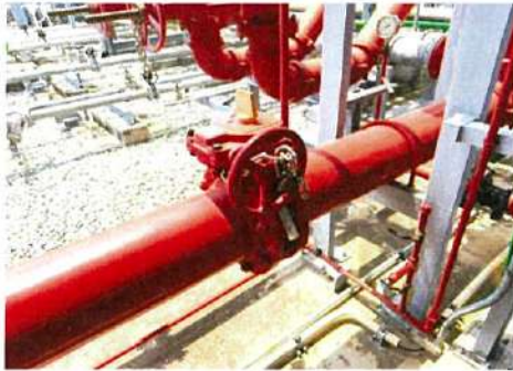
Test pipeline control valve
