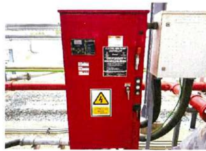
Fire pump controller
